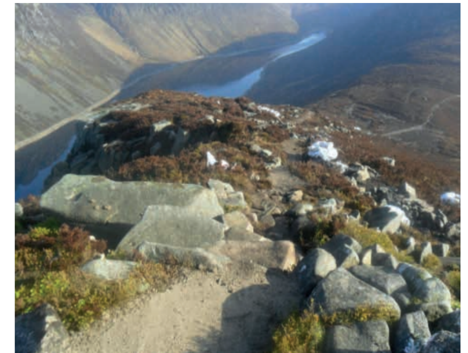
Upland Path Works on Binnian Mountain
